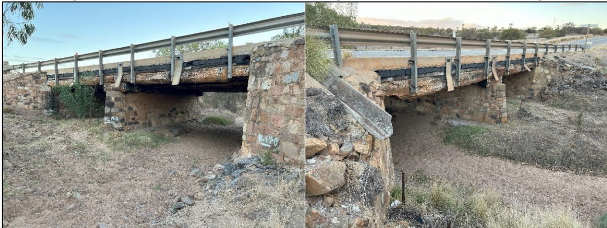
Figure 10.1.3.5 – West (left) and East (right) elevations of Buller bridge
