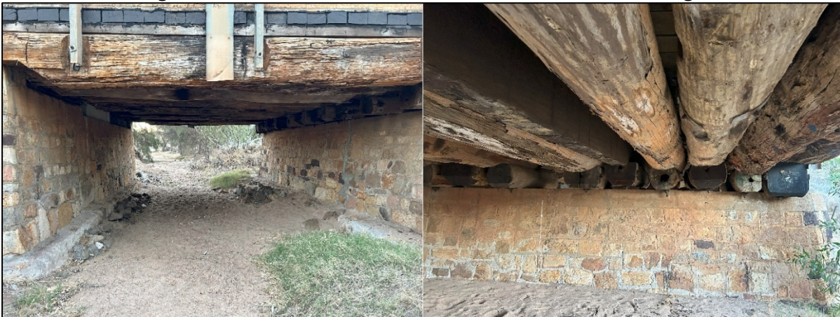
Figure 10.1.3.6 – View of timber underside of Buller bridge
