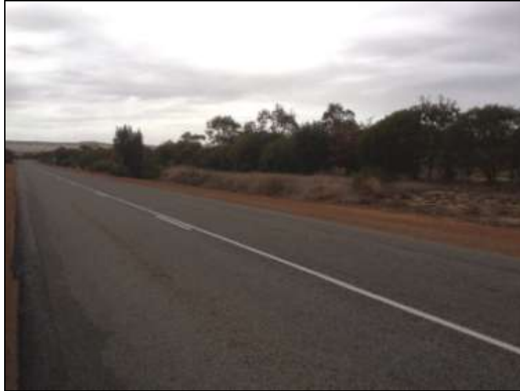
Figure 4 – View of road frontage of Lot 122 Chapman Valley Road looking North
