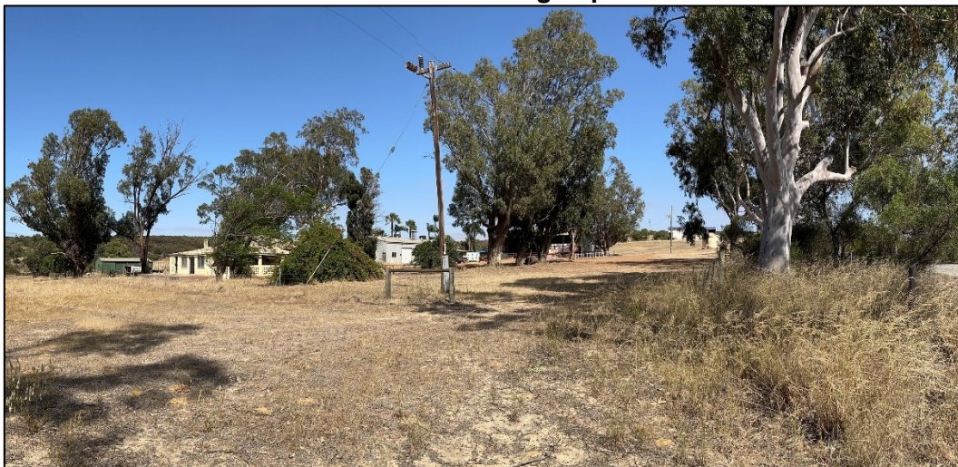
Figure 10.1.1.5 – View of main cluster of buildings upon Lot 14 Nanson-Howatharra Rd
