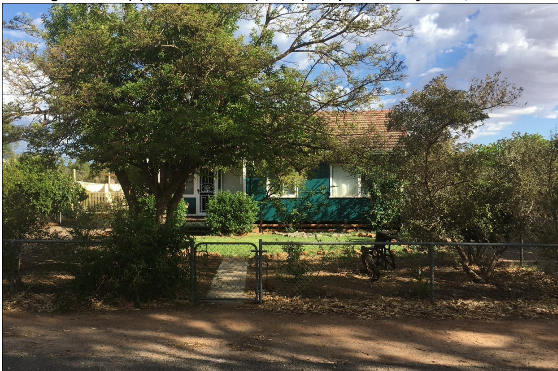
Figure 10.1.1(c) – View of 3287 (Lot 18) Chapman Valley Road, Nabawa
