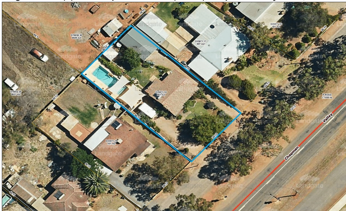
Figure 10.1.1(b) – Aerial photo of 3287 (Lot 18) Chapman Valley Road, Nabawa
