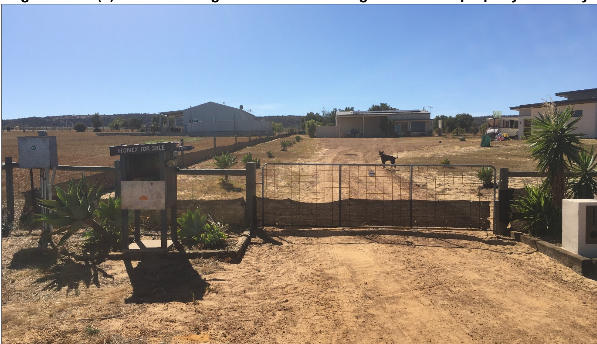
Figure 10.1.2(d) – View looking south-east from road at Lot 274 existing built form
