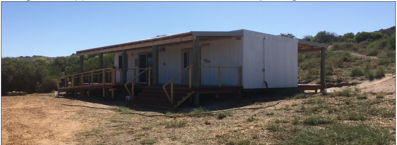
Figure 10.1.1(c) – View of under construction office/shop/manager's residence
