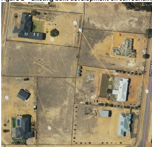
Figure 2 – existing built development on surrounding lots.
