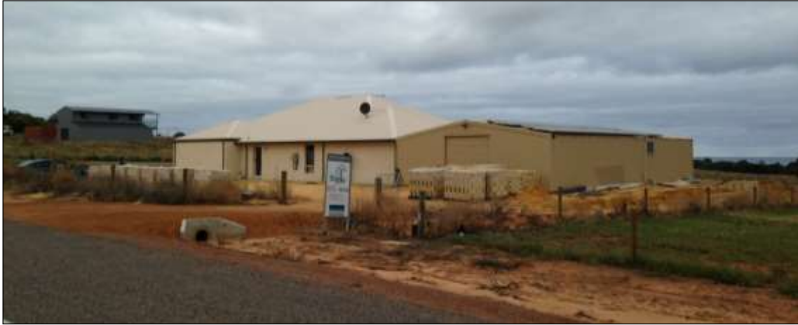
Above: Looking south west from David Road
