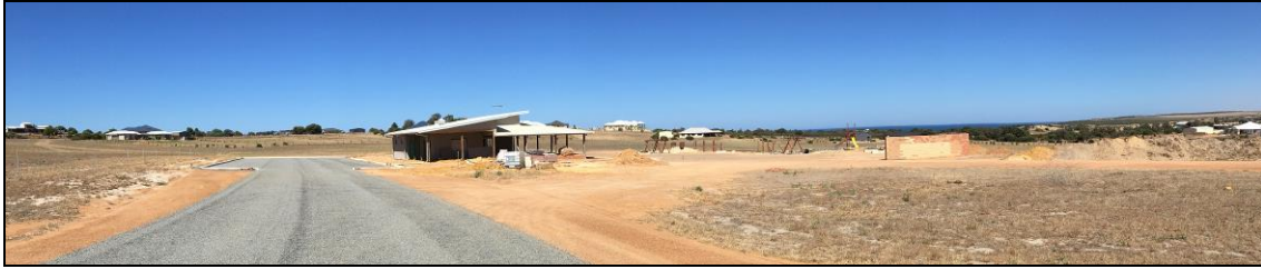
Figure 10.1.4(a) – View looking south-west across Bill Hemsley Park construction site
