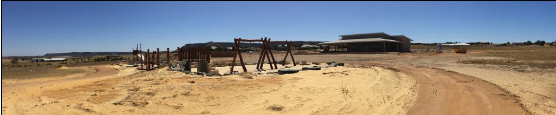
Figure 10.1.4(b) – View looking north-east across Bill Hemsley Park construction site
