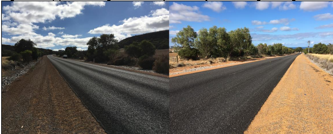
Figure 10.1.5(d) – view along Lot 1455 Chapman Valley Road frontage looking east/west
