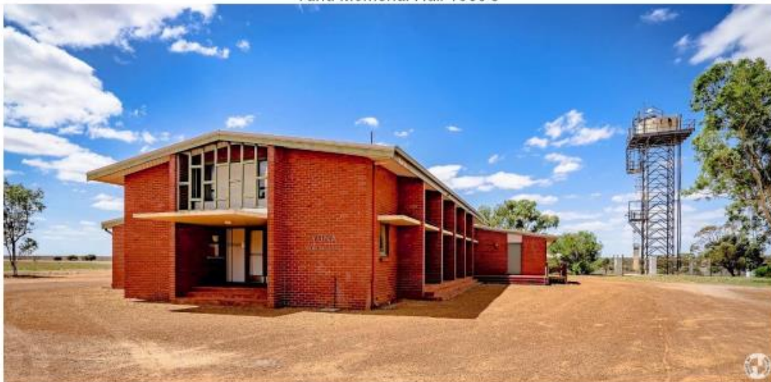
Yuna Memorial Hall photo by Greg Davies
