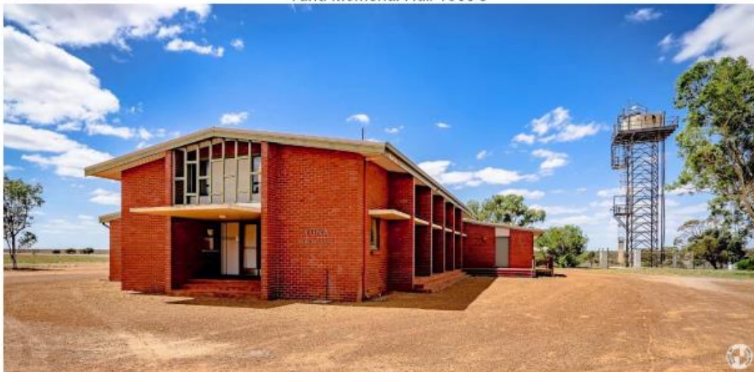
Yuna Memorial Hall photo by Greg Davies
