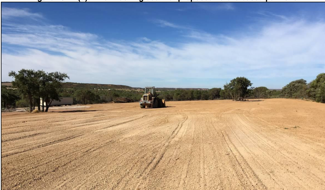
Figure 10.1.1(e) – View looking east at ablation facility placed on-site
