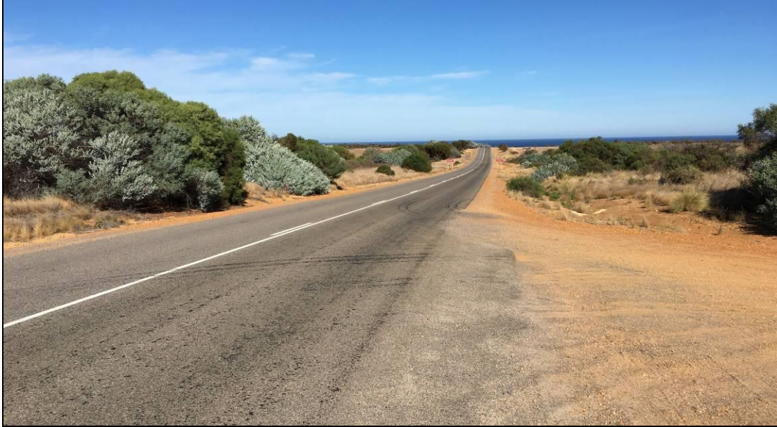
Figure 10.1.2(e) – View west along Coronation Beach Road from access point to Lot 171
