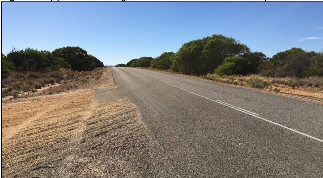
Figure 10.1.2(d) – View east along Coronation Beach Road from access point to Lot 171
