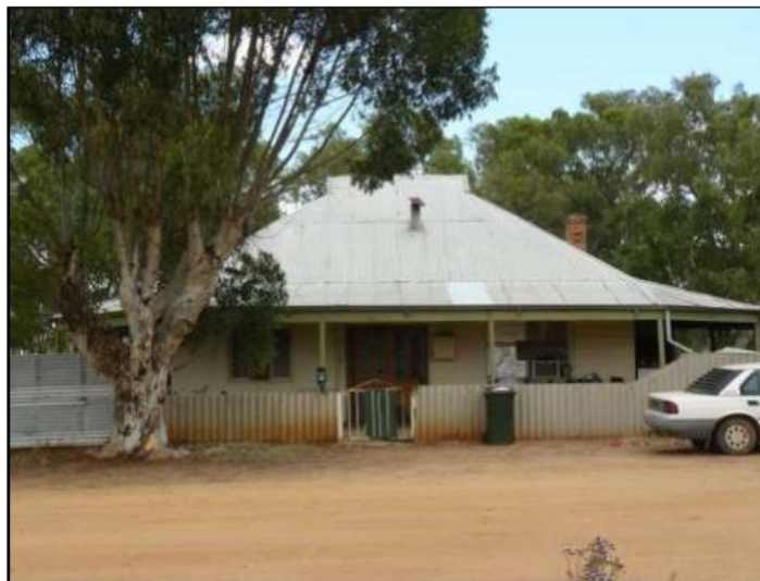
Description: Front facade facing east
