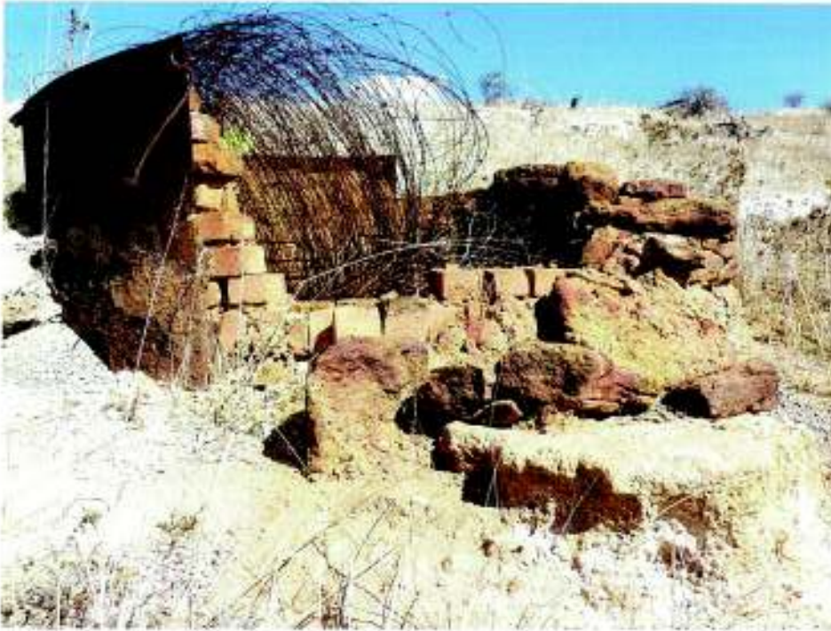
P13670 Lime Kilns, Howatharra Kiln 1: view showing detail of east side. L Gray 15 April 2010
