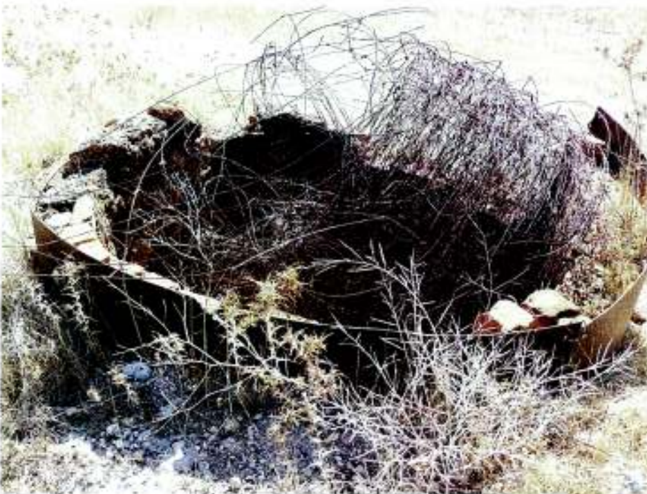
P13670 Lime Kilns, Howatharra Kiln 1: view looking into the kiln from southwest. L Gray 15 April 2010
