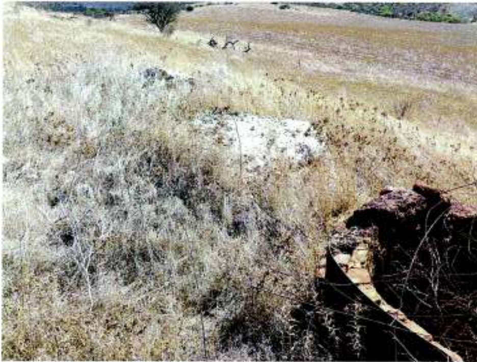
P13670 Lime Kilns, Howatharra Kiln 1: northeast view showing concrete remnant on north side of kiln. L Gray 15 April 2010
