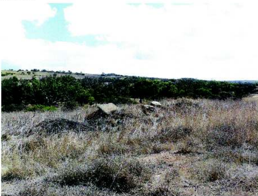
View looking northwest from White Peak Road, showing remnant material (most likely not railway associated) on the east side of the railway alignment, within cleared land. April 2010.
