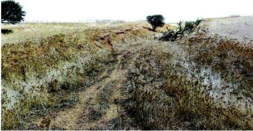
NORTH of the SUBJECT AREA. View several hundred metres north from the intersection of Olsen and Oakajee Roads showing the railway formation. April 2010
