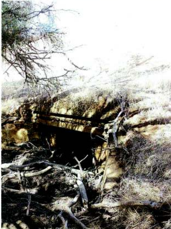
NORTH of the SUBJECT AREA. The culvert in the formation. April 2010
