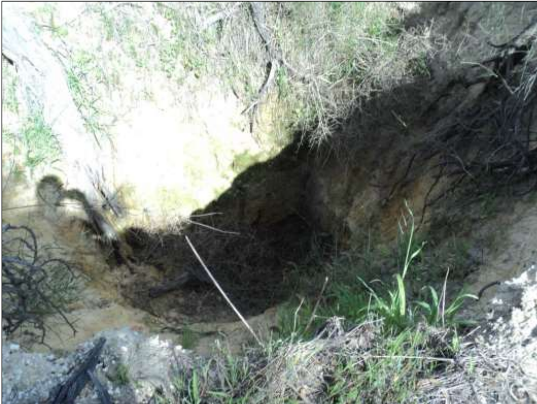
Figure 8 – Well Site upon Reserve 17216 Protheroe Road, Nabawa
