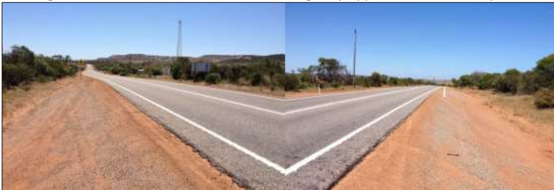
Figure 5 – View of northern and southern highway approaches to access point
