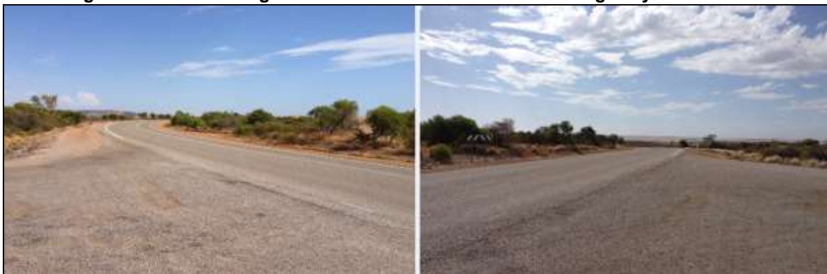
Figure 6 – View looking south and north from ‘Wells Road’ highway intersection
