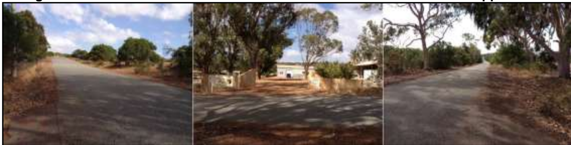
Figure 3 – View of entrance to business and Nanson-Howatharra Road approaches
